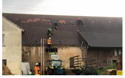
Some slates blown down from the roof on the north side of the building. DI Roofs, DoD1 (<20% loss ratio): IF0+ / F0T1.
