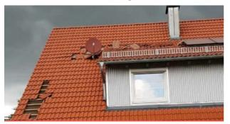
Some slates blown down from the roof on the north side of the building. DI Roofs, DoD1 (<20% loss ratio): IF0+ / F0T1.
