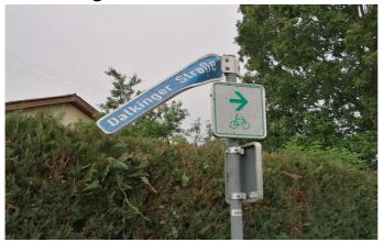
Damage very likely not caused by wind force, but by falling tree or large branches.
