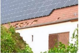
Some slates blown down from the roof on the north side of the building. DI Roofs, DoD1 (<20% loss ratio): IF0+ / F0T1.
